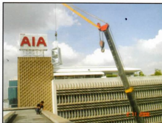
AIA TOWER (THAILAND)
